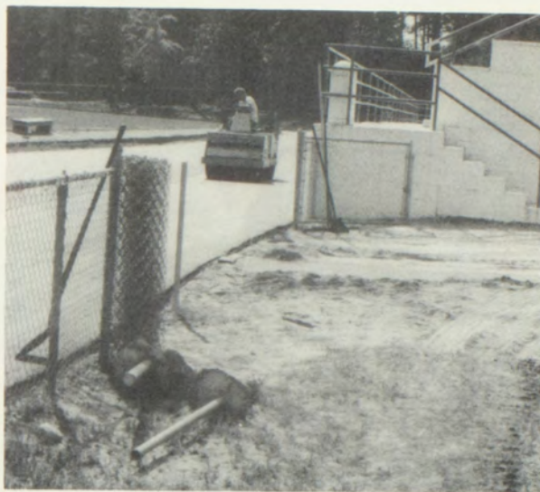
PAVING THE WAY. Putting the finishing touches on the base of the new track, Mr. Bob Shleben of Widdis Sand and Gravel steamrolls the asphalt to prepare it for the rubberized surface. Widdis Sand and Gravel, along with many other local businesses, made substantial donations to help pay for the $80,000 track. Photo by Kari French.
